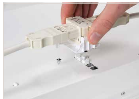
Align the T-connector with the square cutouts.
